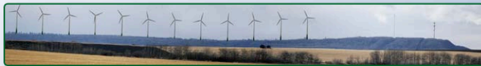
Design concept of Bear Mountain Wind Park near Dawson Creek, B.C. (under construction). Credit: Aeolis Wind Power Corp.
